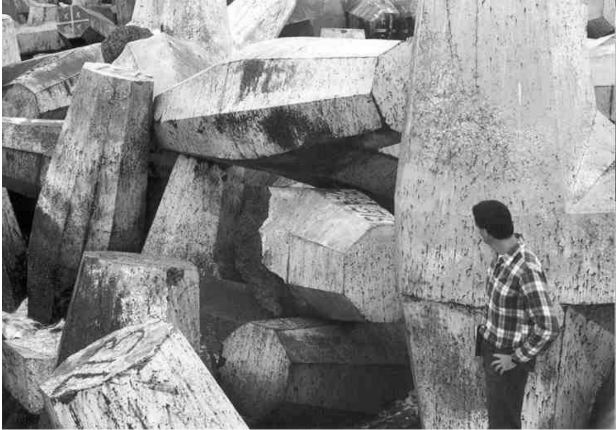
Figure VI-8-1. Dolos breakage on Crescent City, California, breakwater
