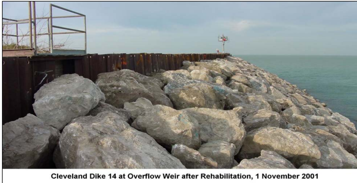
Figure VI-8-9. Cleveland dike 14 after rehabilitation
